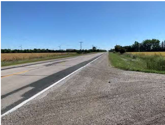
Photo 39: View of municipal road and associated disturbances, facing east
