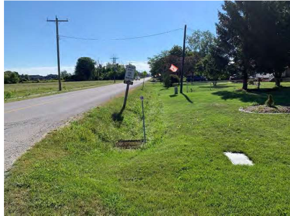
Photo 10: View of municipal road and associated disturbances, facing southeast
