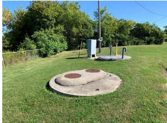
Photo 22: View of existing disturbance, facing northeast
