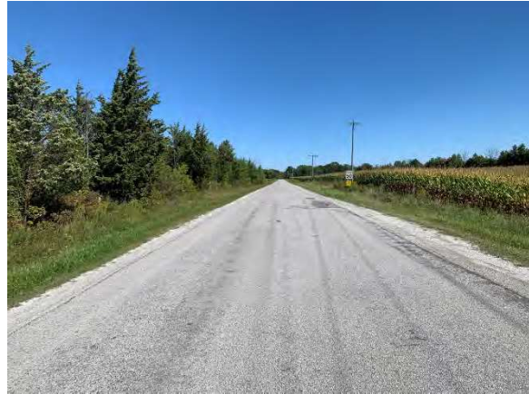
Photo 34: View of municipal road and associated disturbances, facing north
