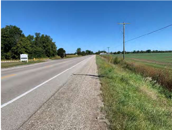
Photo 29: View of municipal road and associated disturbances, facing north
