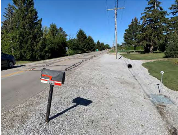
Photo 13: View of municipal road and associated disturbances, facing northwest
