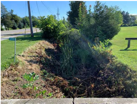
Photo 1: View of municipal ditching, facing northeast
