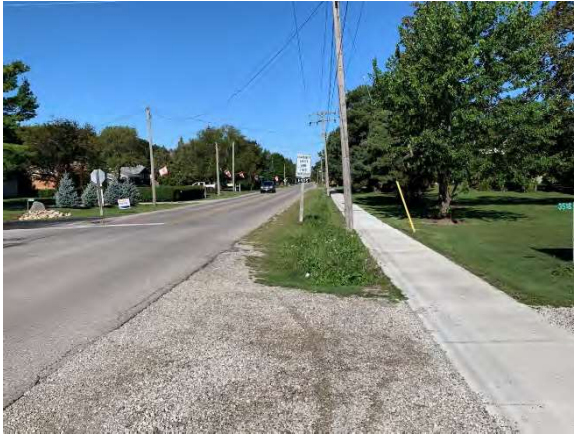
Photo 9: View of municipal road and associated disturbances, facing northwest
