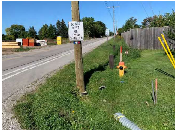
Photo 12: View of municipal road and associated disturbances, facing northwest
