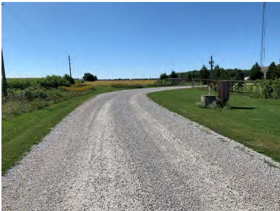
Photo 43: View of existing laneway and associated disturbances, facing southwest
