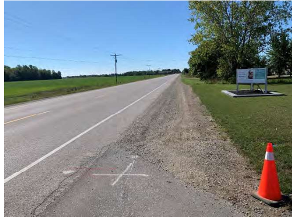
Photo 30: View of municipal road and associated disturbances, facing south
