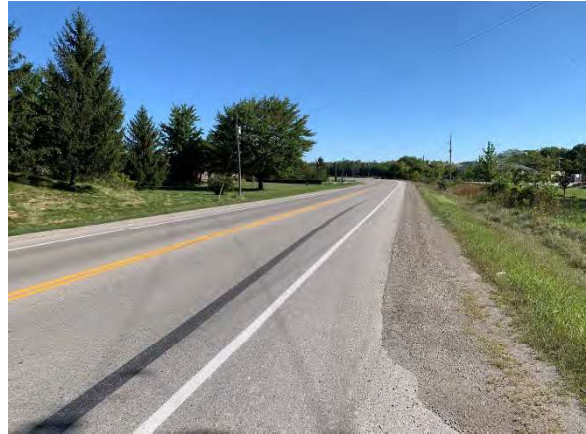
Photo 18: View of municipal road and associated disturbances, facing northeast
