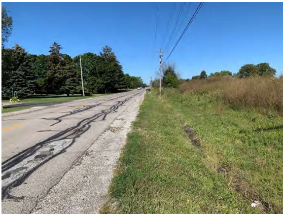
Photo 15: View of municipal road and associated disturbances, facing northwest
