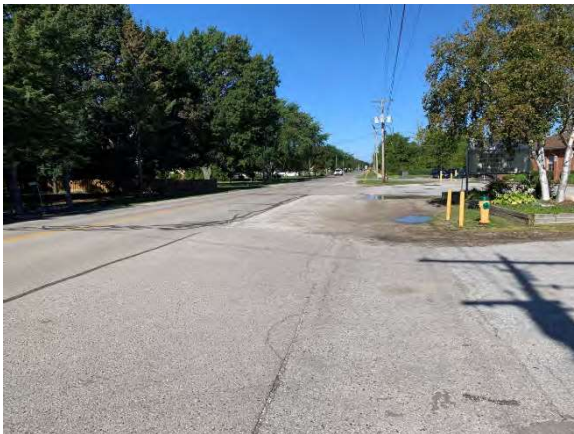
Photo 11: View of municipal road and associated disturbances, facing northwest
