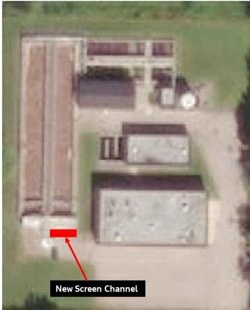
Figure 8-4. Wyoming WWTP Screening Upgrades
