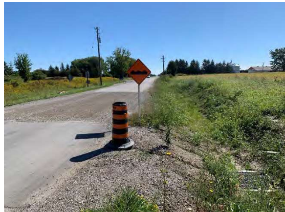
Photo 32: View of municipal road and associated disturbances, facing east
