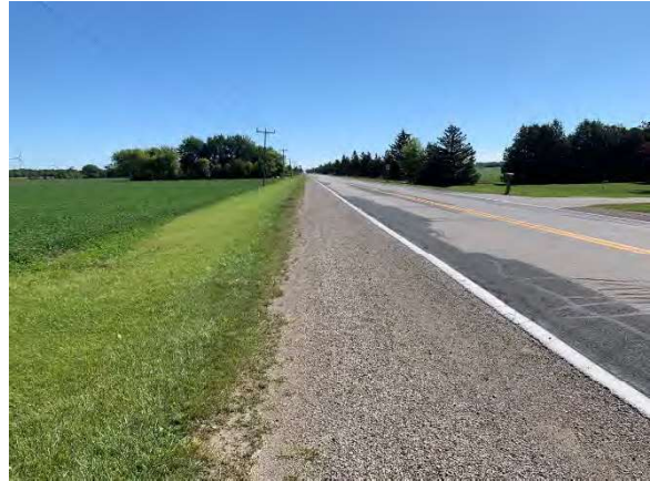
Photo 38: View of municipal road and associated disturbances, facing east
