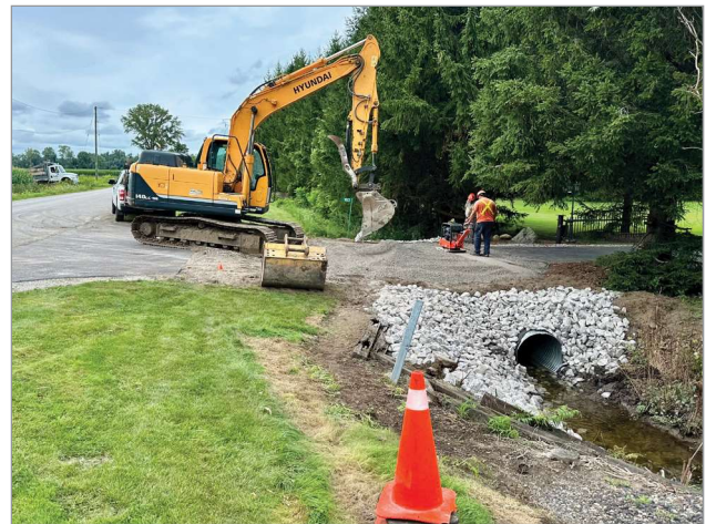
Figure 2. A drain maintenance project.
